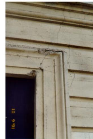
B. Cracking at corner of entryway to stadium in Section A (north side of stadium).
