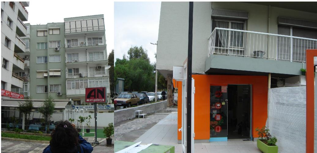
Figure 6.9: Examples of tilted houses in Karşıyaka due to soft fundament of the houses. The pictures were taken during the field trip in autumn 2006.
