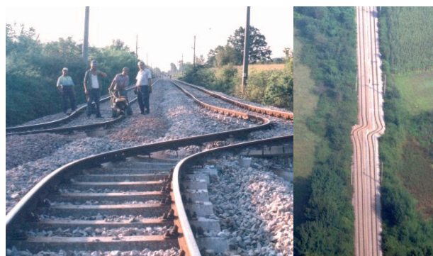
The picture shows a strike-slip fault rupture, which displaces the railway line. The pictures are taken in connection with the earthquake in Izmit, Turkey, on August 17, 1999.
