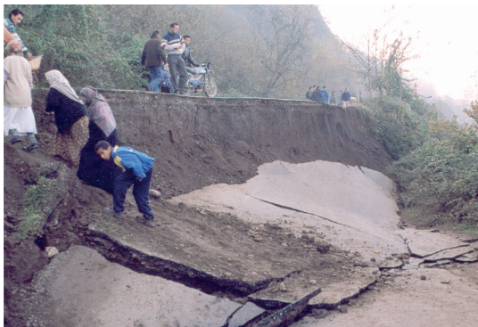
The picture shows a normal fault in connection with a destructive earthquake in November 1999, close to the city of Düzce, Turkey.
