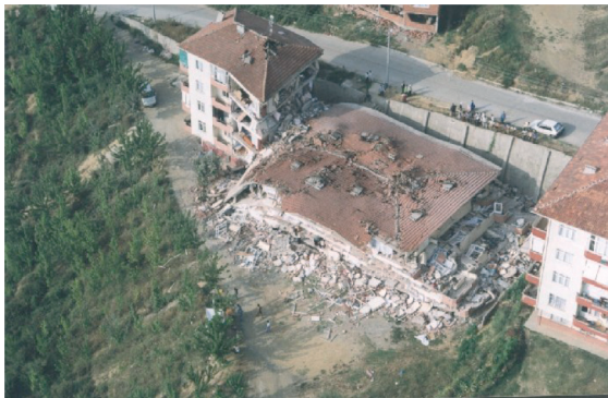
The pictures show the buildings that collapsed in connection with the catastrophic earthquake in Izmit, Turkey in 1999. Much of the damage was the result of bad construction practices.
